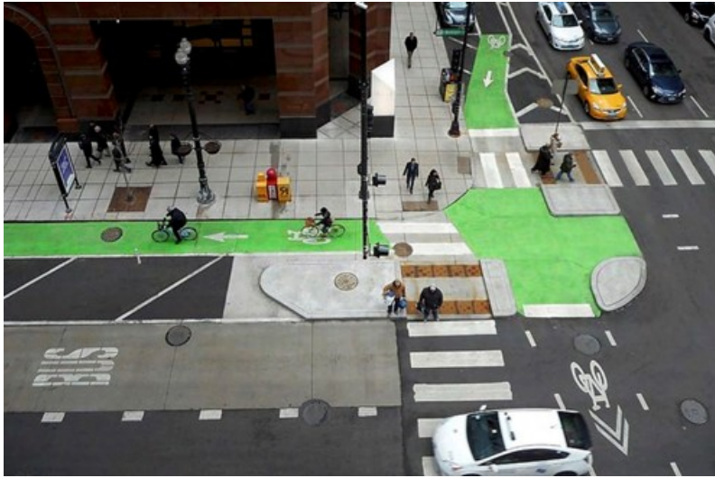
A protected intersection in Chicago. Photo: Chicago Department of Transportation (Bike Program)/Brian Almdale
